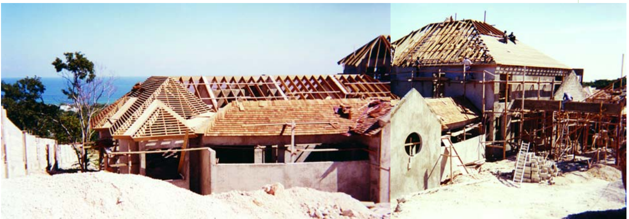
The roof is finally going on — time to plan the party.
